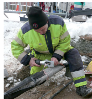
Crimping with Elpress crimp tool PVL611.
