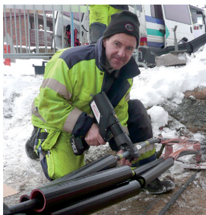
Crimping with Elpress crimp tool PVL1300.
