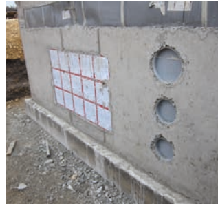
ZVR 150/300 and ZVR 200/300 concreted next to HSI 150
