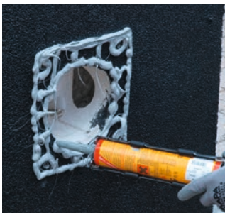
wall surface prepared with Sikaflex
