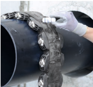
GKD 400 – preparation of installation with lubricant GM
