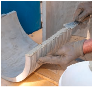
FZR-G 350/300 with filler of installation set Z-FZR-G
