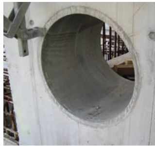
FZR 400/300 installation in sewage plant
