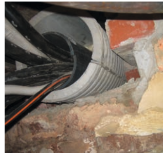
FZR-G 150/350 refurbishment within brick-built wall
