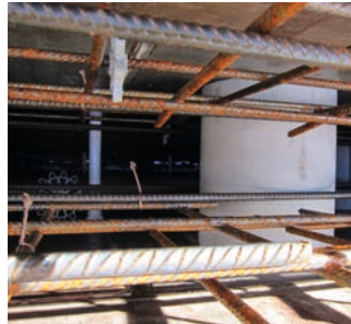
ZVR 200/300 installed in formwork
