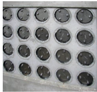
FZR 100/240 sealing pipe route
