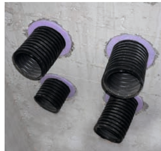
view inside of the building (insulation rings)
