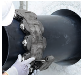
GKD 400 – installation of segments
