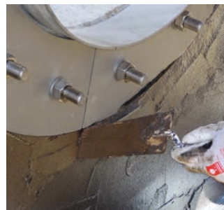
HRD 300-FUF/300 stainless steel design with connection to PMBC by fleece inlay, see page 37
