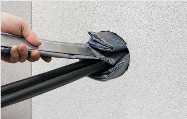
S 90 retrofitting for core drillings and wall sleeves with a HRD
