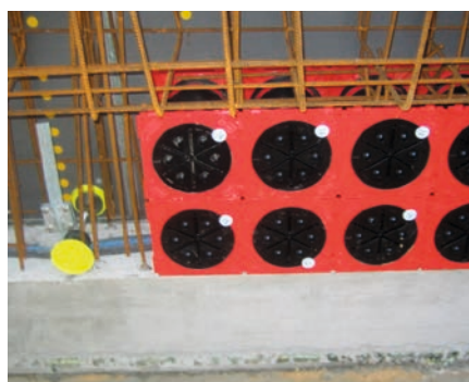
HEA-PK-M12/240 with the PE protective covers fixed at the formwork with nails next to the cable entry HSI 150.
