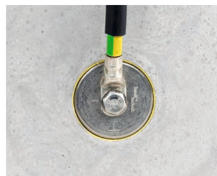
HEA-IS-M12 after the installation. The earthing connection with a cable lug and the contact plate is visible.
